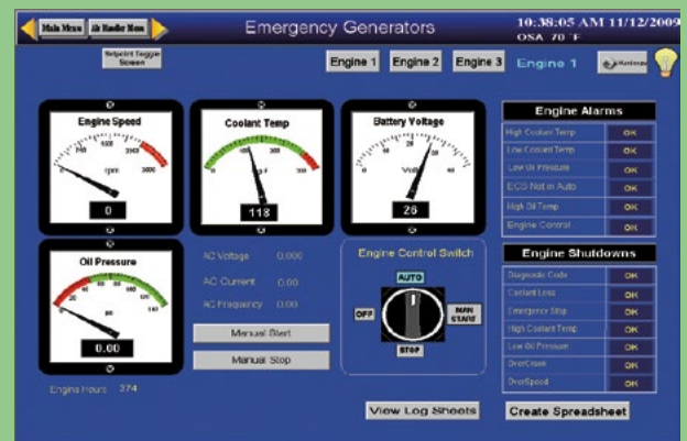
View of Emergency Generators
