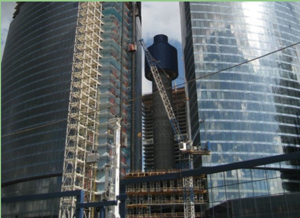
The Federation Tower Under Construction Moscow, Russia
